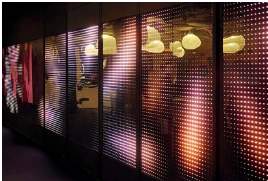
The 50m-long video graphic wall, which consists of 37mm resolution LED pixels
