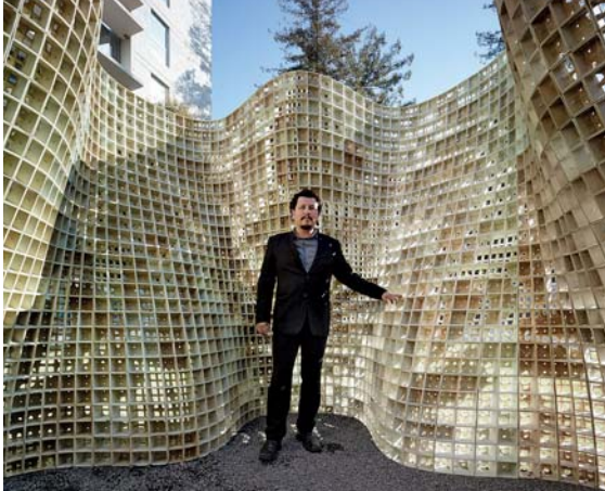
Bloom, a freestanding 3D-printed cement pavilion, is made of 840 customised blocks
