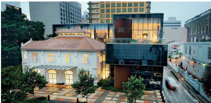
WOHA's Space Asia Hub consists of two conserved historic buildings joined by a contemporary glass infill structure
